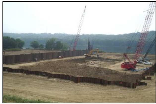
Figure 17: Sheet Pile Installation
