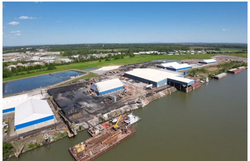
Figure 1: Existing Fiver Rivers Terminal
