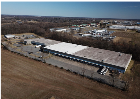
6001 Lindsey Rd | East Loomis Armored US, LLC leased 50,000 SF of industrial space
